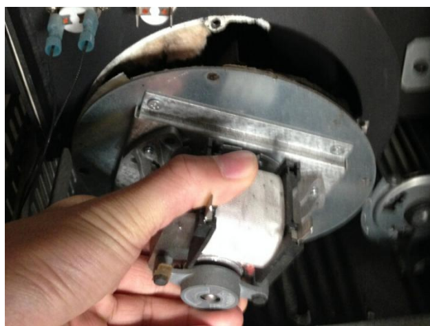
Figure 37: Remove combustion motor and clean
